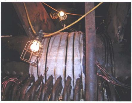
**6. Precision bore.** Two tube bores were precision-machined for the new tube-to-header connections. *Courtesy: Thielsch Engineering Inc.*
